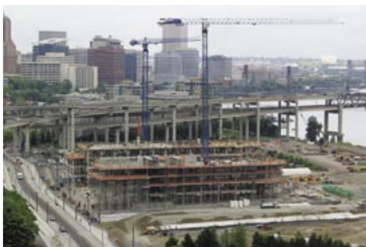
View of current building construction.
