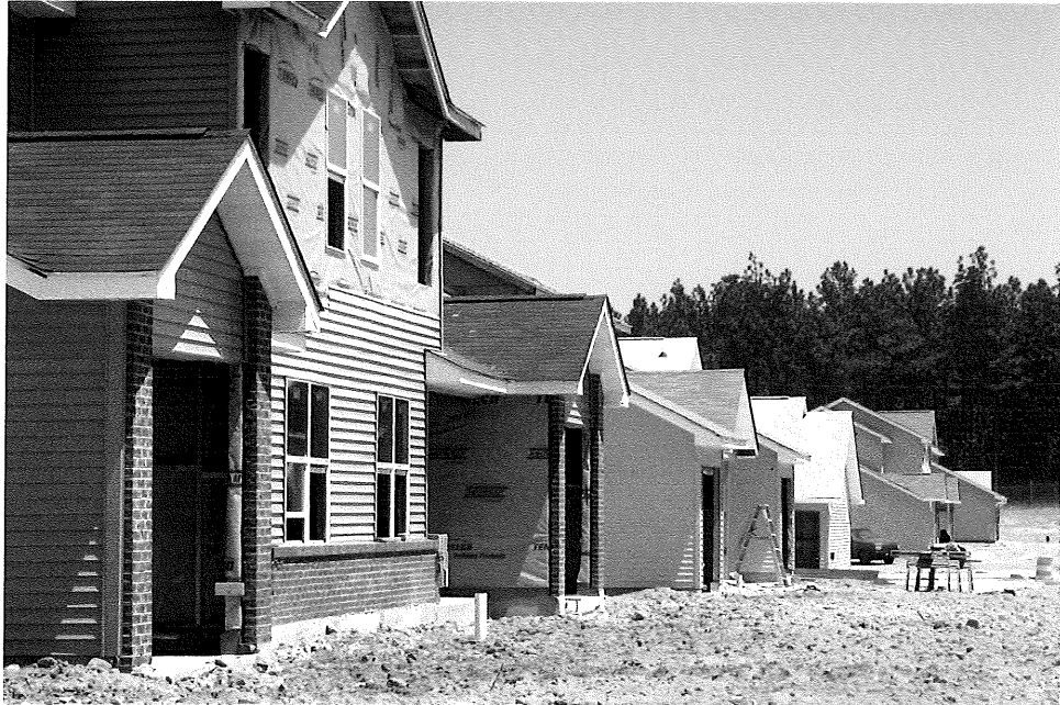
Figure 1. Building houses converts high value salmon habitat into areas suitable for family living, but unsuitable for salmon. (Source: U.S. Army Corps of Engineers.)
